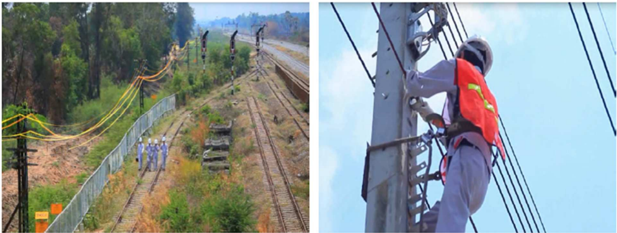
Figure 5: ITEL EPC business included fiber roll out and data center
